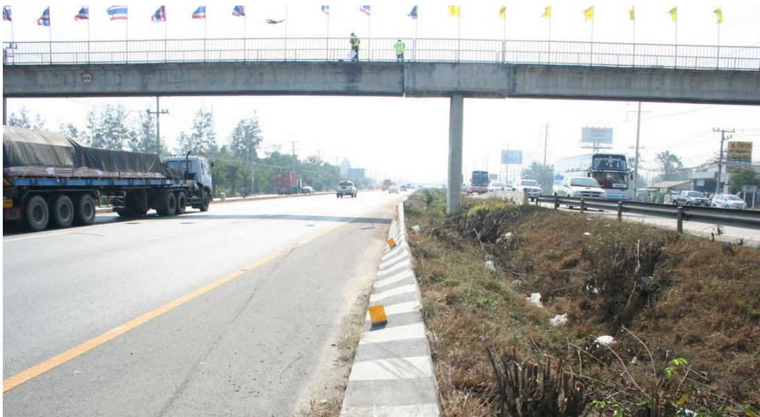
Figure 3-11: Approach Concrete Barrier
