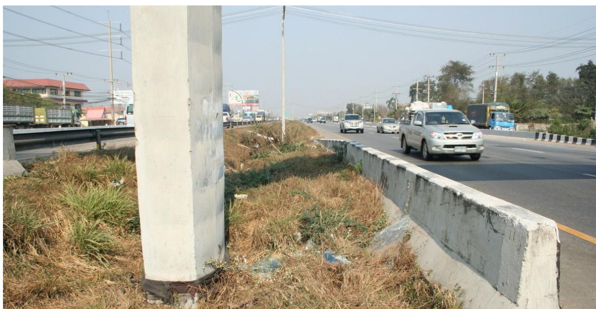
Figure 3-9: Pedestrian Bridge Column at the Depressed Median
